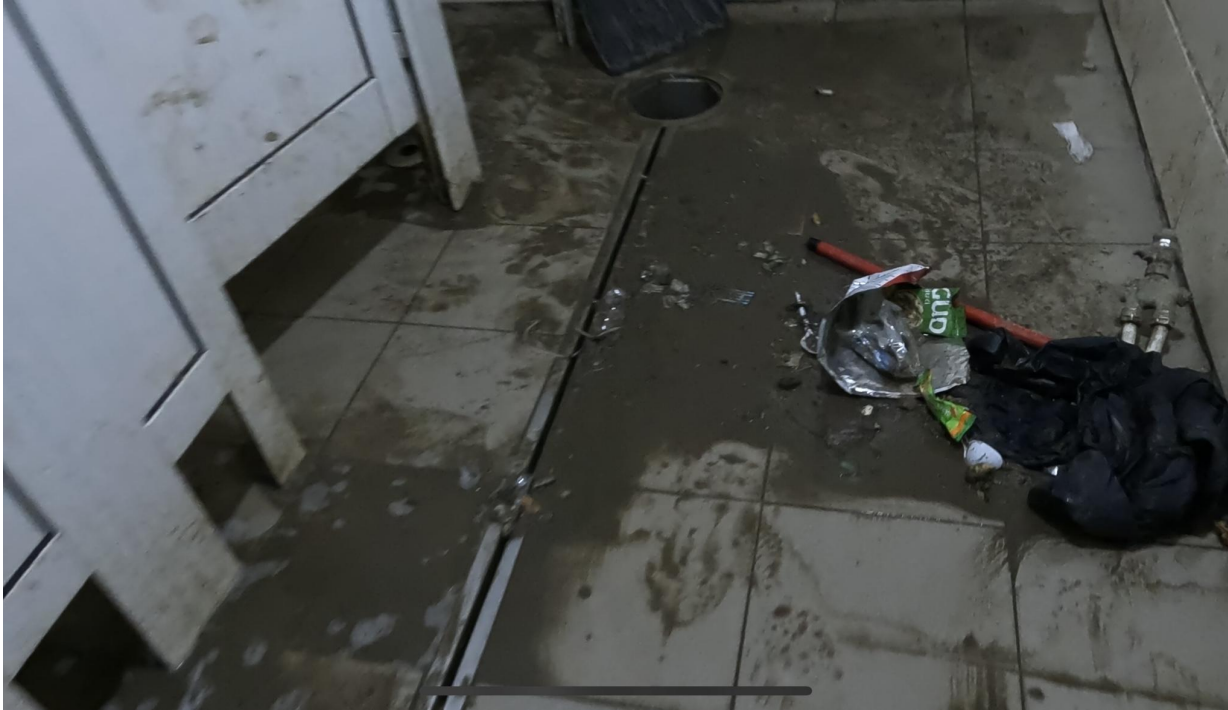
Subotica Camp, 10th January 2023, floor in shared bathroom, 03:00
